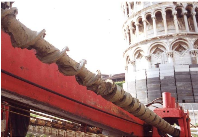
Fig. 25. The underexcavation
