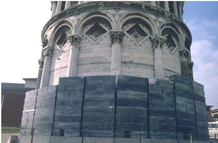
Fig. 21. The provisional intervention by lead ingots counterweight
